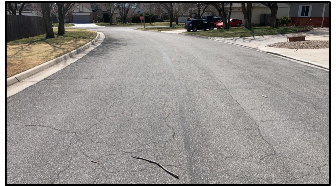
TIGHT or SEALED CRACKING
