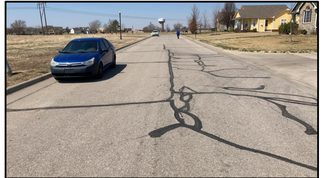
TIGHT or SEALED CRACKING
