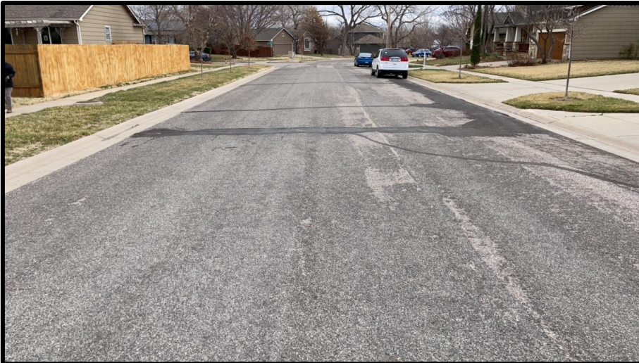
SEALCOATED or CRACKED SEALCOATED BUT BEGINNING TO SHOW SIGNS OF DISTRESS
