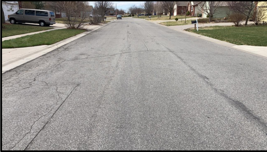
SEALCOATED or CRACKED SEALCOATED BUT BEGINNING TO SHOW SIGNS OF DISTRESS
