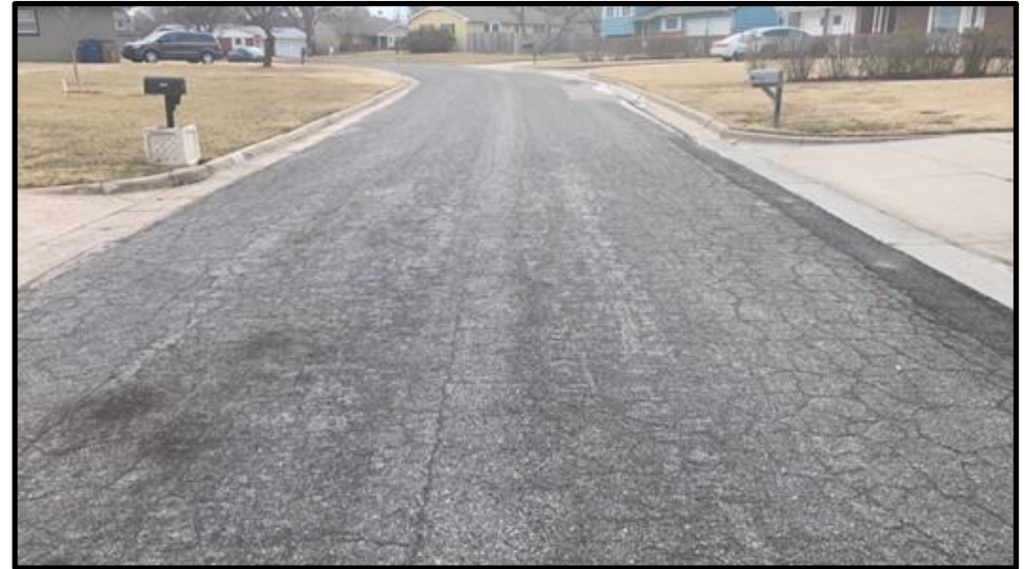
EXTENSIVE BLOCK CRACKING
